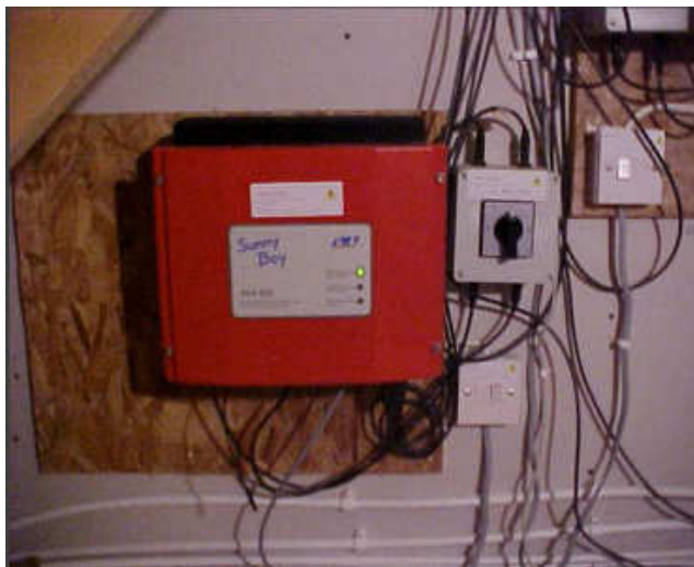
Image 2: Improper wiring method
