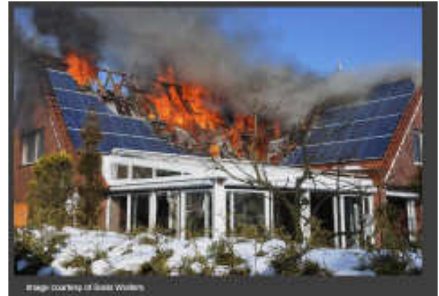
Image 1: Owners should stay away from the PV system during and after a fire and inform the fire brigade about the particular hazards from the PV system.
