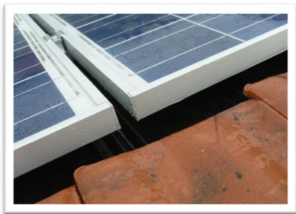
Figure 2. BAPV installation. The Modules are installed on top of the existing roof
