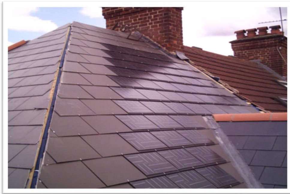
Figure 17. Sunslates. Compatible with large Swiss Eternit slate. Source: Solsticeenergy
