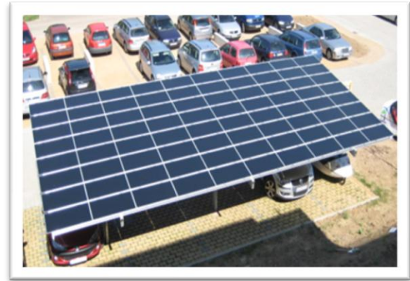
Figure 6. Car Shelter based on thin film technology. In the future, these elements will be used for the charging of electrical vehicles (First Solar)
