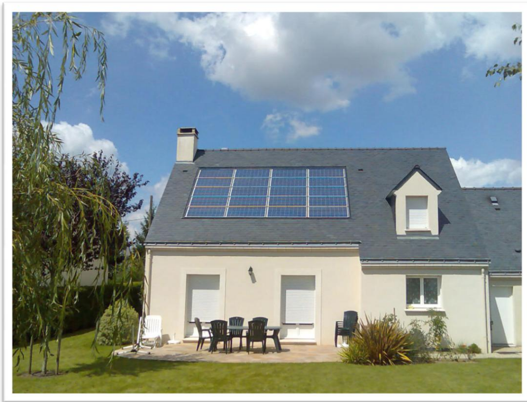
Figure 10. Oryon. Waterproofing system using standard laminated PV modules allowing an esthetical integration and optimal performance. Source: Solstis
