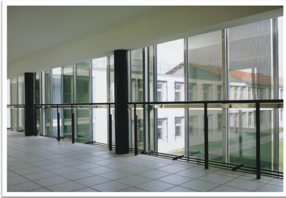
Figure 13. Semi-transparent facade based on Thin Film technology (Source : Schott Solar )
