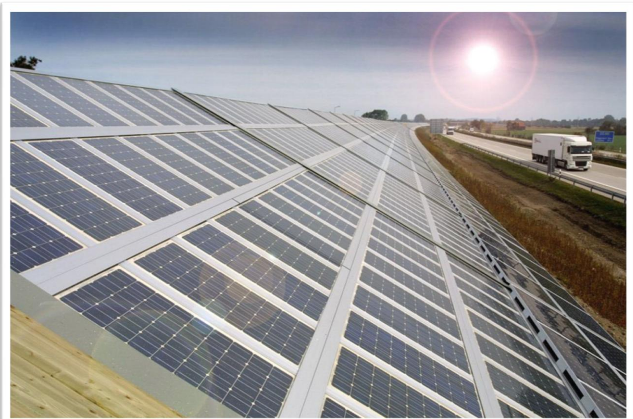
Figure 7. The 500kWp sound-barrier with ceramic based PV modules installed next to the Munich airport (Isofoton)
