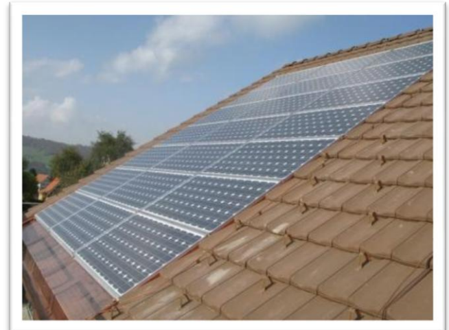
Figure 5. Fastened BIPV system on a pitch roof. This system allows a simple and quick assembly of the modules. It is a system meant for aslope roofs and requires an impermeable roof covering that has to end in the eave (Schüco)
